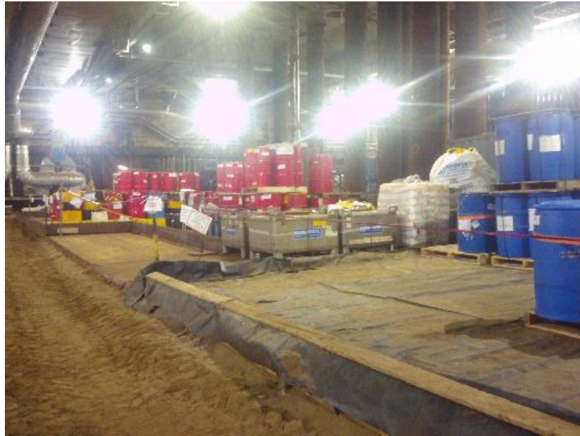
Photo 5. Temporary secondary containment for chemical storage in the Core (planned for upgrade)
