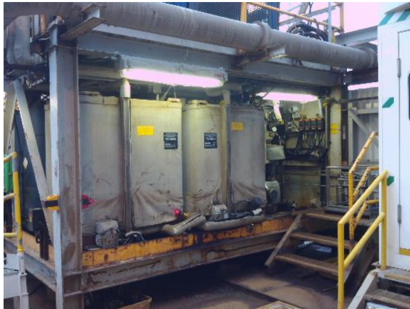
Photo 4. Chemical injection skid (secondary containment planned for renovation)
