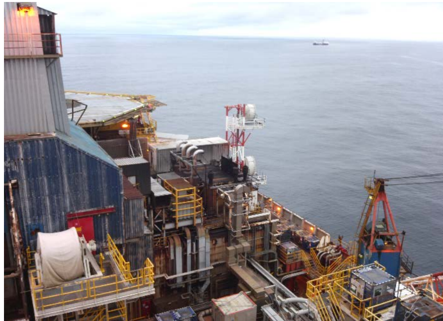
Photo 1. PA-A Platform (general view including drilling rig and helideck)
