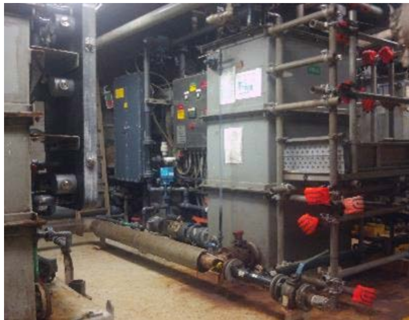
Photo 6. Sewage Treatment Plant (one of three units on-board PA-A)
