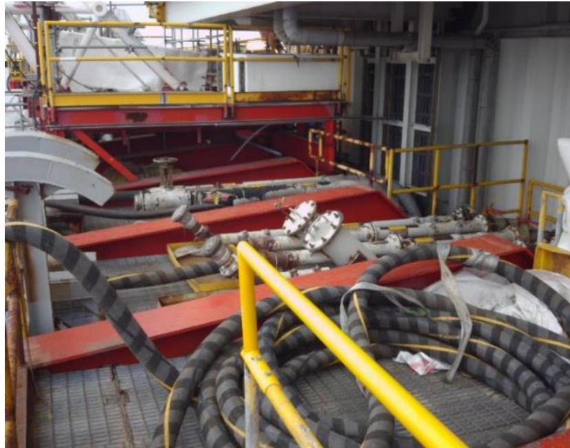
Photo 7. Bunkering point for diesel fuel and OBM (provided with secondary containment system and drip trays)
