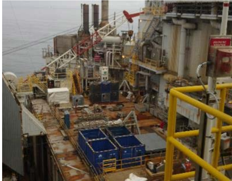
Photo 3. Deck areas (including deck crane) with WHRU in background
