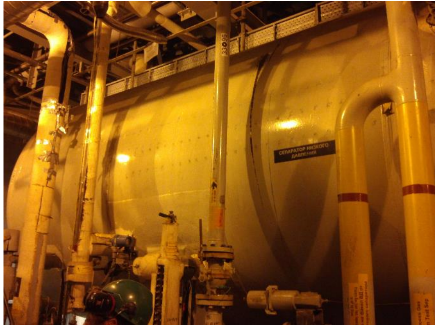
Photo 9. Low pressure separator in Process Module (part of 3-phase process)
