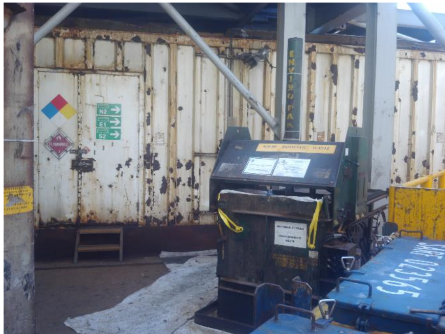
Photo 13. Waste compactor (deck)
