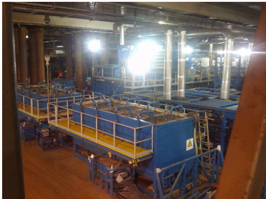
Photo 14. Contractor operated 'Frack and Pack' plant located in Core
