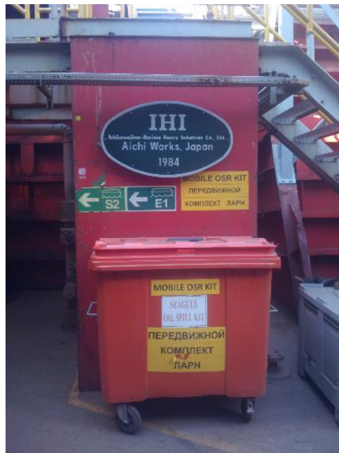
Photo 10. Example of multiple local oil spill response kits present in deck and process areas (well signed and well stocked)
