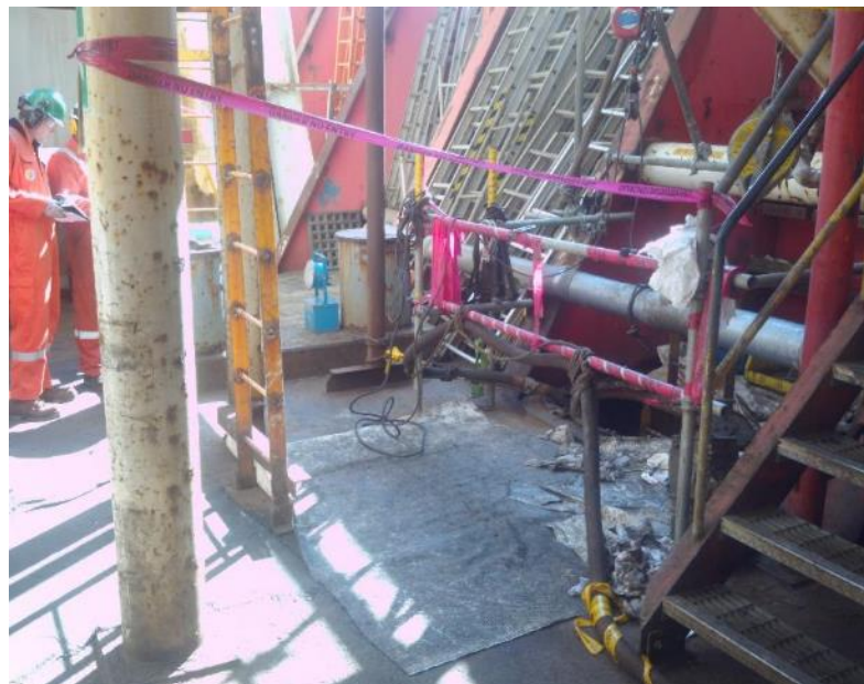
Photo 8. Cordoned work area for OBM tank clean-out and inspection (trip hazards were noted – temporary hose and absorbent matting)
